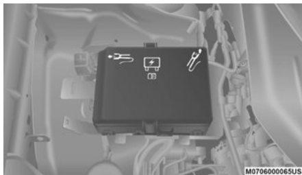
Front Power Distribution Center
