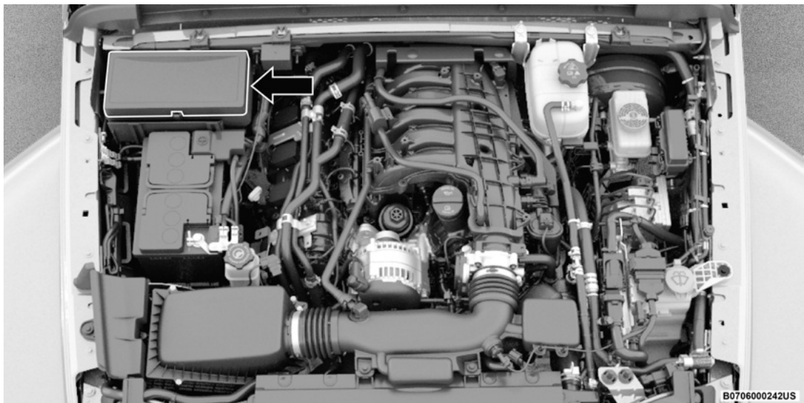
Power Distribution Center Location
