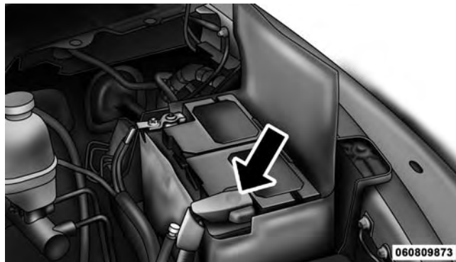
Positive Battery Post
