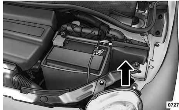
Front Distribution Unit
