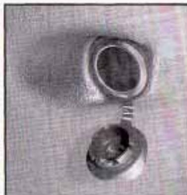
Remove the tethered cap to use the outlet. When not using the outlet, be sure to cover it with the protective cap.
