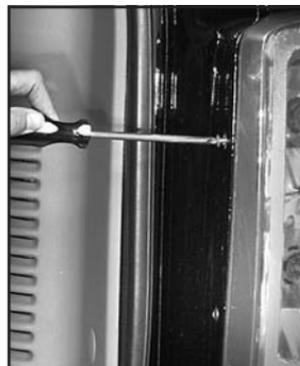
1. Use a screwdriver to remove the two screws from the lamp assembly.
