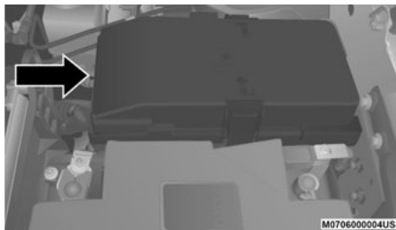
Power Distribution Center
