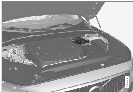
The 12 V support battery is located in a box next to the spring strut in the engine compartment.
