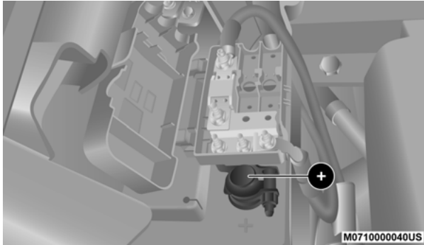
Positive Battery Post
